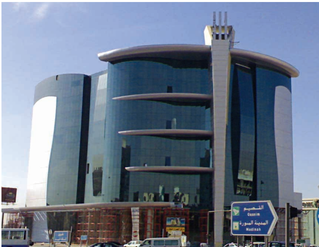
An office building in Riyadh, Saudi Arabia, utilizes the world's first curtain wall system, which secures the glass panels to the exterior of the building.
